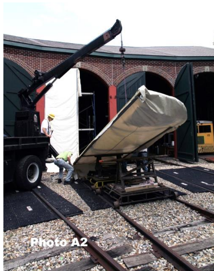
Photo 2 – Shows the door being lifted to an upright position.
