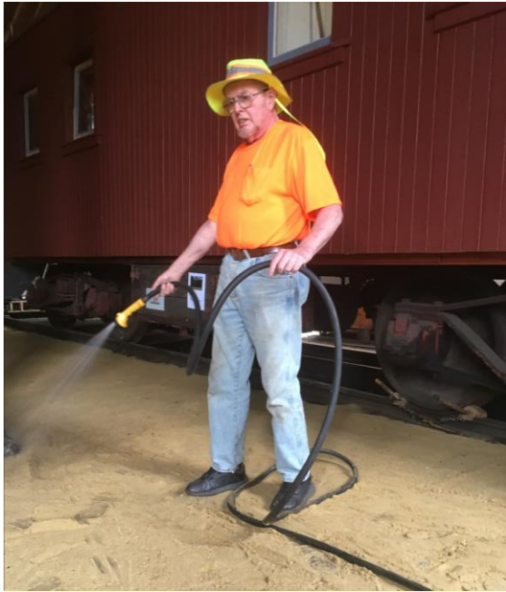
Rolf Johnson seen here watering his luscious new lawn... Not really... He's wetting down the sand between pits 1 and 2 in the roundhouse before compaction. See page 3 for Roundhouse Floor. (Bob Hassett Photo)
