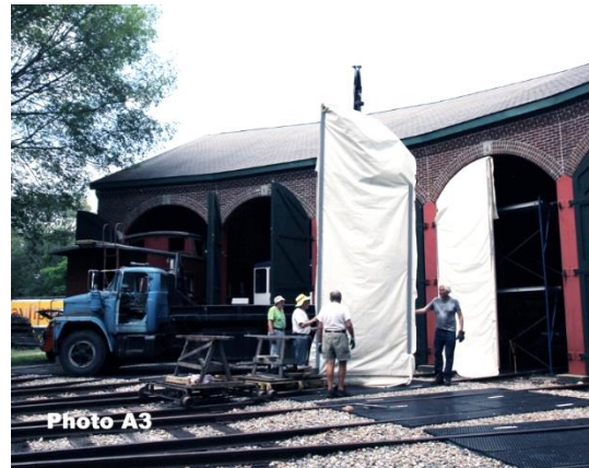
Photo 3 – Shows the door being moved towards the door opening.
