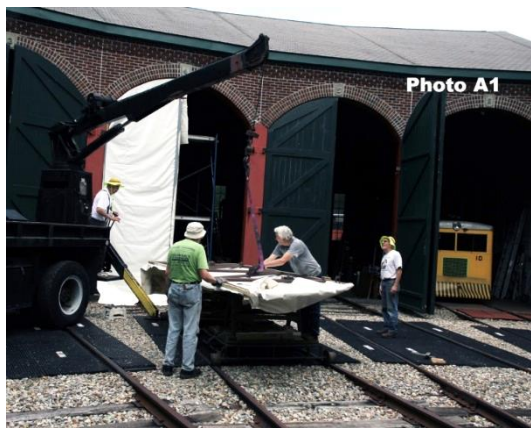
Photo 1 – Shows the belts being applied so the door could be lifted into position.
