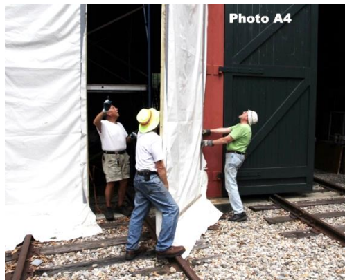
Photo 4 – Shows door being lowered onto the door pins.
