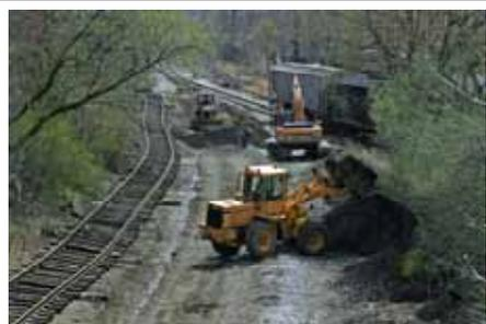
With tracks and ties on left, numerous pieces of equipment are lowering the track grade that passes beneath Rte 66 to allow auto rack trains to pass just outside the museum fences. – R.A. LaMay
