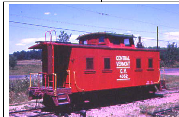
Work will soon commence on the restoration of the CV center cupola caboose #4052. The caboose will be moved into one of the completed tracks inside the roundhouse. Rail will extend outside so when the caboose needs metal-work the caboose can be rolled outside. This photo was taken prior to its move to Willimantic and also before it was damaged by fire. (R.A. LaMay Collection)
