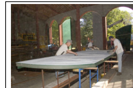
Duke York and Andrew Fischer do maintenance work on the 16' wooden roundhouse doors. (Photo by R.A. LaMay)
