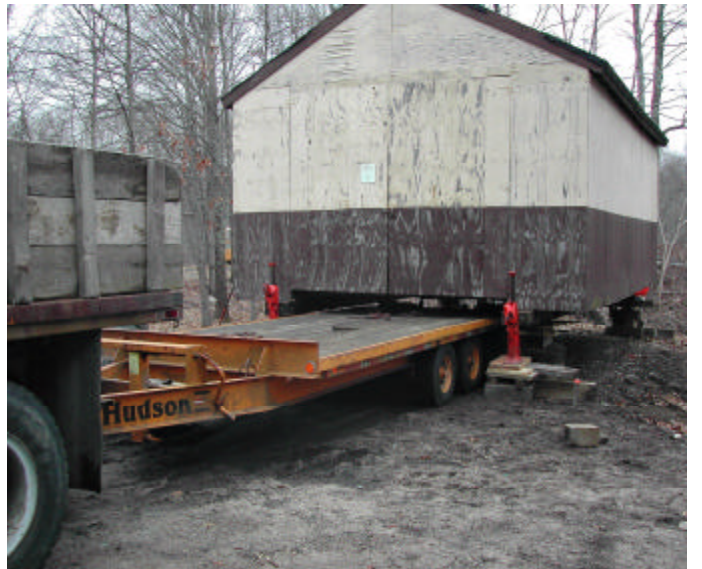
The Rail bus Shed was moved to its new location inside the Columbia Junction Village area. Will be used as a blacksmith shop. – (photo by Robert J. Hassett)
