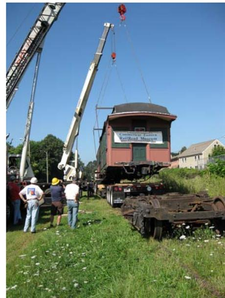
With the car safely suspended by the cranes, the trailer can now be moved and the trucks placed under the car for lift down. (Carolyn Stanich Photo).
