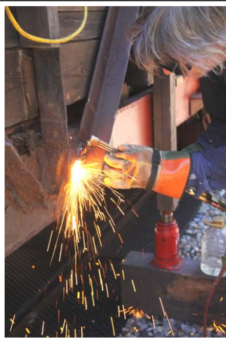
Steve Dolan cuts out a rusted section on the Central Vermont Center Cupola Caboose No. 4052. (Robert A. LaMay Photo)
