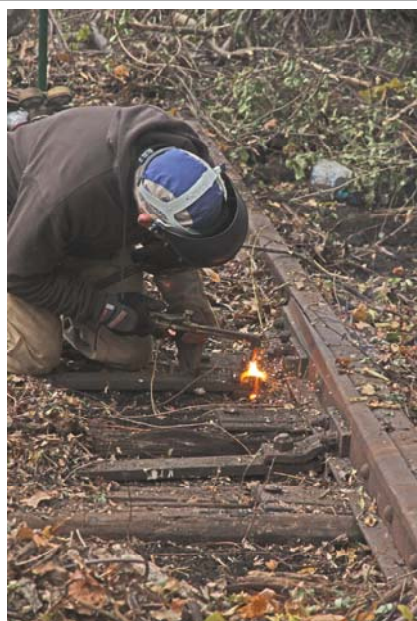
Bob Hassett burns off rusted rail bolts at the rail recovery that took place at Hartford, CT. (Robert A. LaMay Photo)
