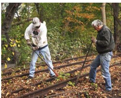
Andy Fischer and Art Hall, Jr. pull up old spikes from rail taken at the rail recovery project at Hartford, CT. (RA LaMay Photo)
