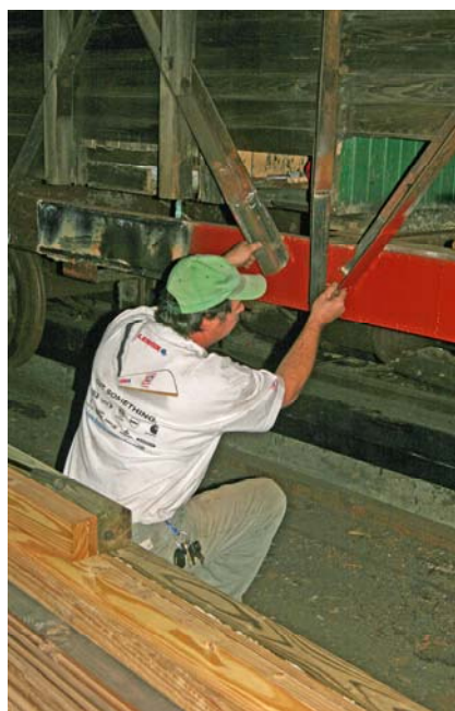
Bill Voorvaart continues to work on the restoration of the CV no. 4052 caboose. (Robert A. LaMay Photo)
