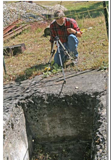
Mark Granville does some close measuring for the next track project which will see another track set along next to the ash-pit. (Robert A. LaMay photo)
