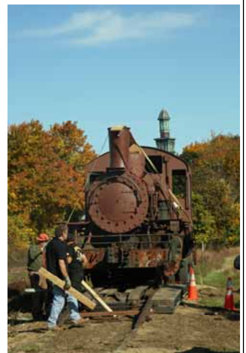
Many hands make light work as Steam 10 is prepped to be off-loaded in the Bridge St. Yard. (Robert A. LaMay Photo)
