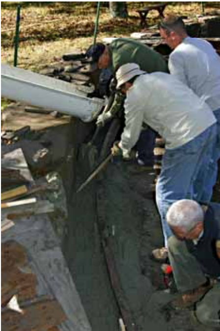
Dick Arnold, Adam Bycholski, Rolf Johnson, and Bob Hassett help move the fresh concrete into position under the ring rail. (Robert A. LaMay Photo)
