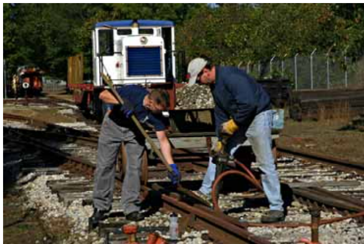
Track Work – one of our favorite pass times. Here Adam Bycholski places ballast into position so Andy Fischer can tamp in down. The museum's 25 ton switcher 'Lil Tugger' sits in the background. (Robert A. LaMay Photo)
