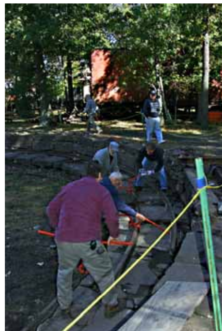
This photo shows various members moving the ring rail into position in the turntable pit. (Robert A. LaMay Photo)
