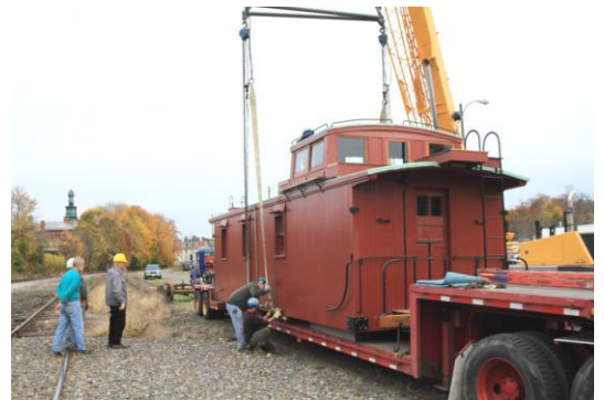
Dick Arnold along with others observes the prep work taking place prior to the caboose being offloaded from the trailer to the railroad trucks. (R. A. LaMay Photo)
