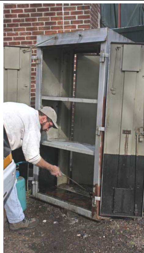
Andy Fischer works on cleaning up the Kendall Spur signal box. (Robert A. LaMay Photo)
