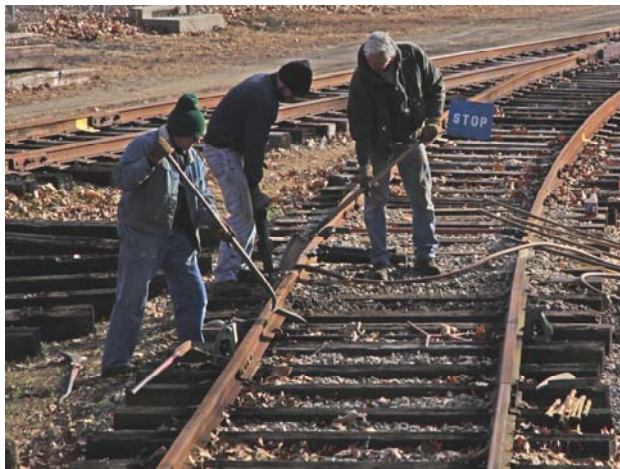
From left to right – Bill Bouchelle, Andy Fischer, and Art Hall, Jr. work replacing some bad ties along the Groton Freight-house siding at Columbia Jct., CT. (Robert A. LaMay Photo)
