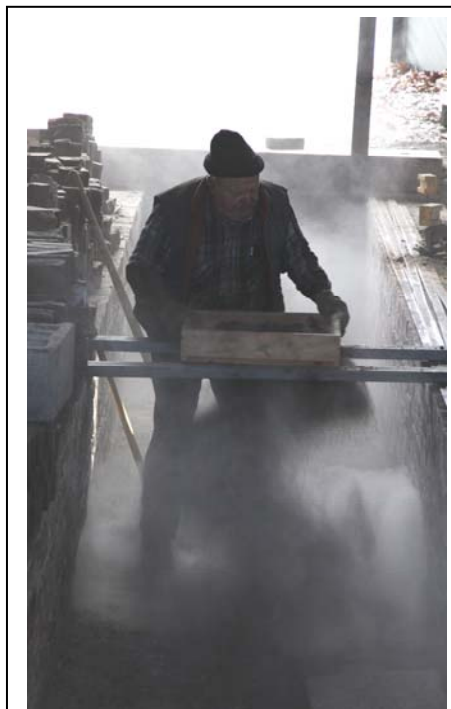
Adrian Atkins sifts gravel to put a base of fine sand along the bottom of Pit number 2. (Robert A. LaMay
