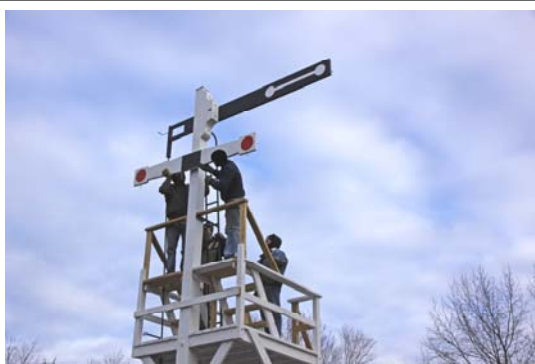
Art Hall, Jr. (upper left) assists Andy Fischer (upper right) align the lower sign board while down below Dick Arnold, lower left and Bill Bouchelle, lower right look on. (Robert A. LaMay Photo)
