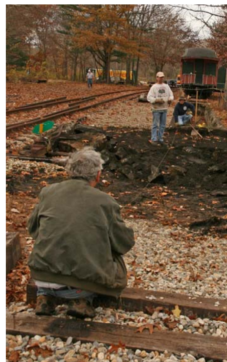
Art Hall, Jr. and Bill Bouchelle hold line as Andrew Fischer verifies its center for Ash-pit track. (Robert A. LaMay Photo)
