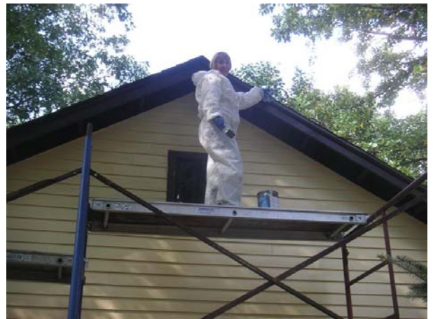
Carolyn Stanich puts finishing touches on the New Haven Railroad Section-house in Columbia Jct. (Robert Hassett Photo)
