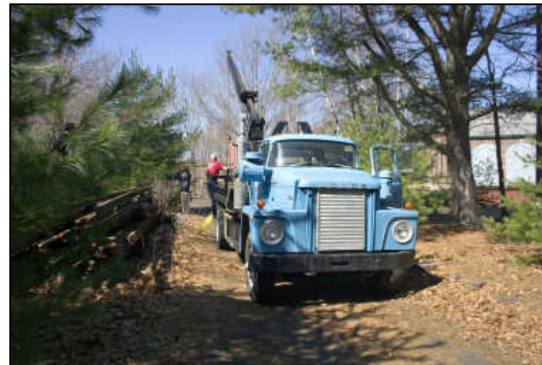
Our new crane truck works to move some rail into the Roundhouse. R.A. LaMay photo
