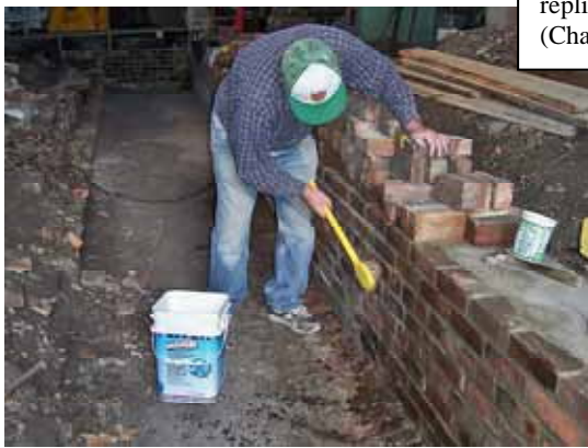
This photo shows John Ference acid washing side walls of Pit no. 2 (Adrian Adkins Photo)
