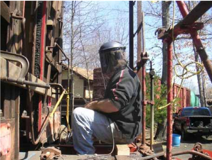
With weather and warm sunshine around the museum a lot of progress is taking place both inside and outside as evidenced by this photo of Bill Voorvaart doing some restoration works on the 4052 caboose. (Robert Hassett Photo)
