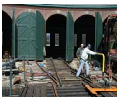
Andy Fischer aligns turntable during the restoration of pit track 4. Note the new progress to the left of Pit 4. (Robert A. LaMay Photo)
