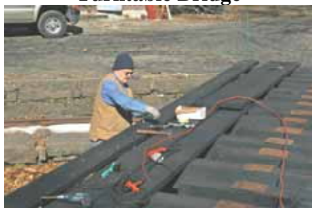
Duke York works on the new planking for the turntable (R. A. LaMay Photo)
