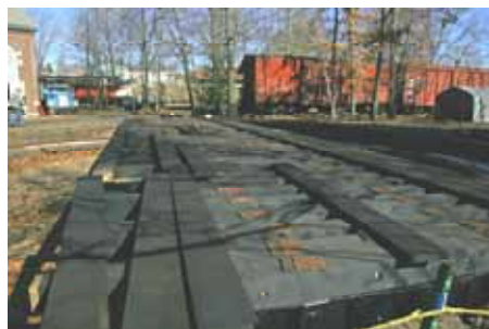
The above view shows completion to date. The planking is just about completed and the rail should go on very shortly. Watch for next issue of GTJ. (Robert A. LaMay Photo)
