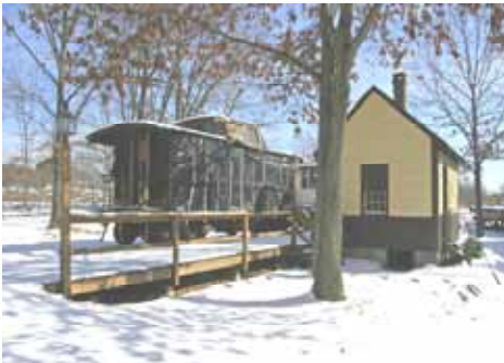
Once the turntable project is completed the next on the restoration lists is the CV #4052 caboose. It will be moved inside the roundhouse where the restoration will begin. (Robert A. LaMay Photo)
