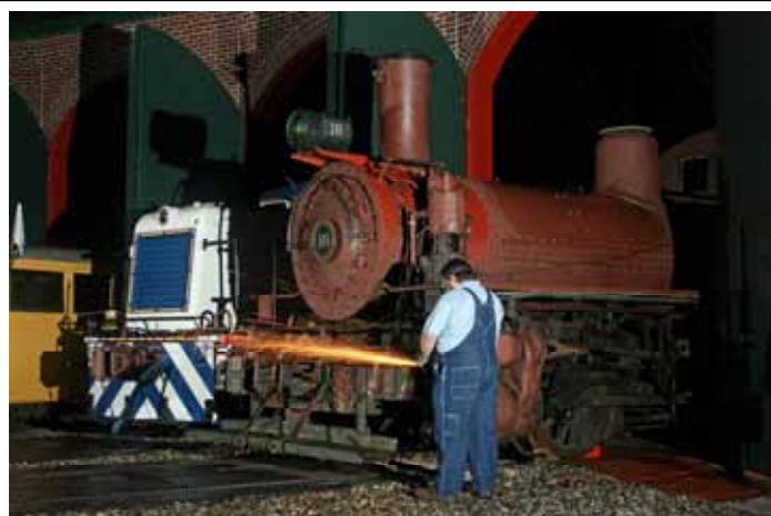
This interesting photo by Nick Palazini shows Rick Cizik hard at work doing some night repair work on Steam No. 10 just outside the Columbia Junction Roundhouse.
