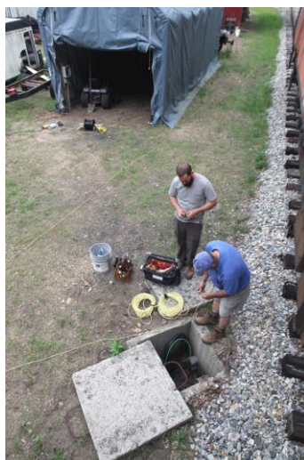
Jim Brennan along with his son Mike installs a new line to the small equipment tent at the museum. (Robert A. LaMay Photo)
