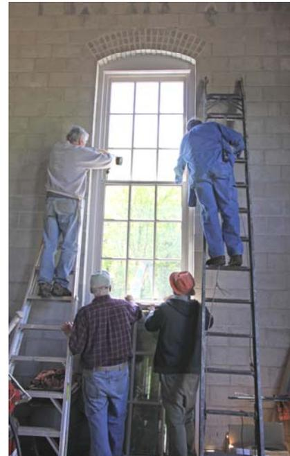
Members work on the interior of the roundhouse installing window hardware so the windows would operate correctly. (Robert A. LaMay Photo)
