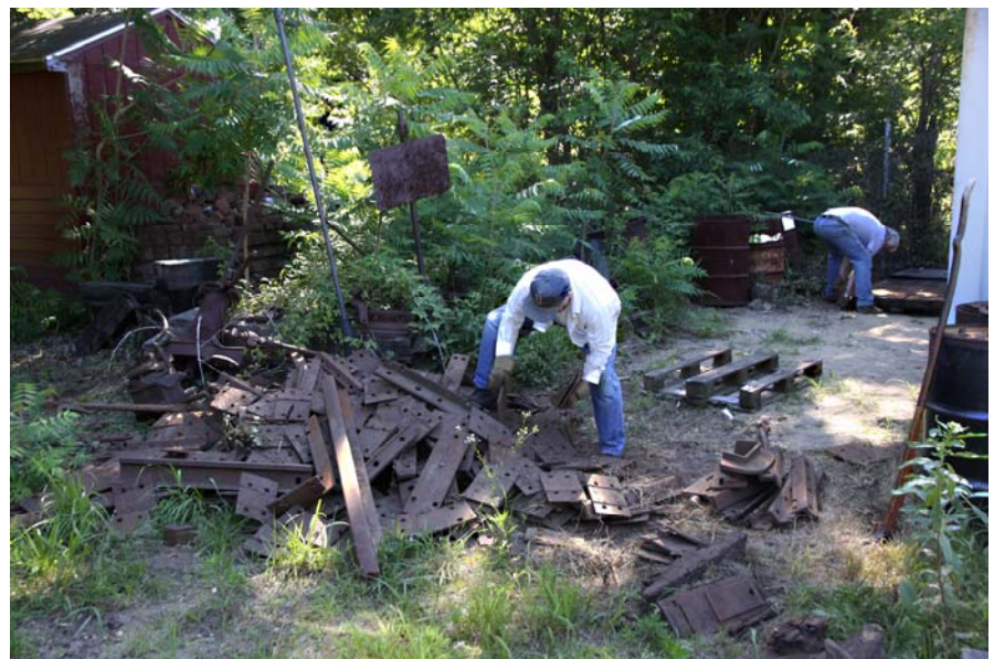
Bill Bouchelle (left) goes through the pile of rail parts and separates good tie plates and joint bars. In the background Art Hall Jr. stacks the good tie plates into manageable stacks for future rail projects at the museum. (Robert A. LaMay Photo)
