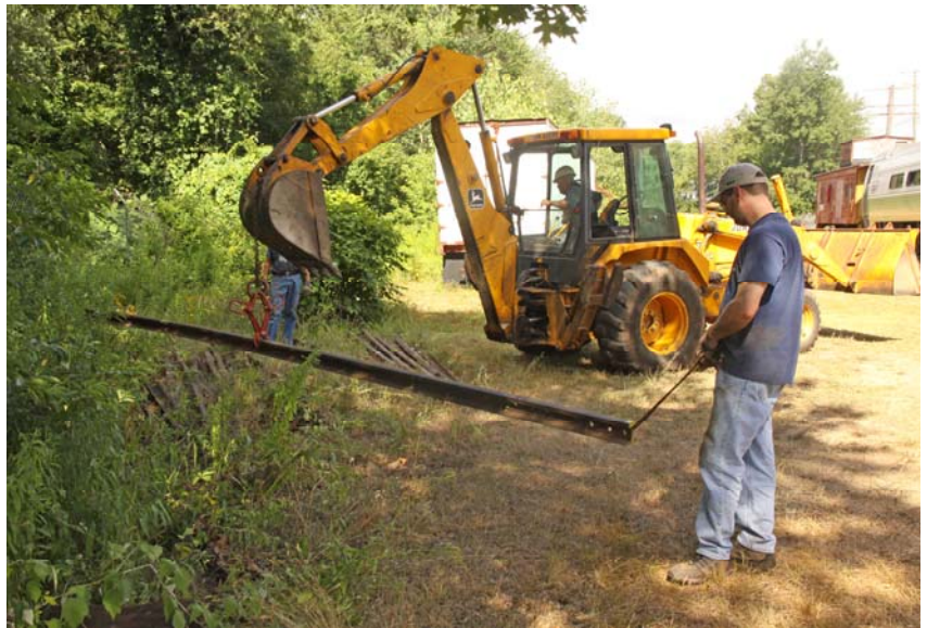
Andy Fischer guides a piece of rail to the proper location while machine operator Adrian Atkins slowly and safely moves the piece of rail. All of the rail in this area is being moved to a central track area. (R.A. LaMay Photo)
