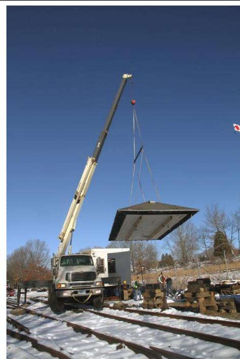
Crane lifts roof of Niantic Railroad Bridge Control House which is being placed on the building behind the crane. Seems we always pick to do these projects in sub-freezing weather. (R.A. LaMay Photo)
