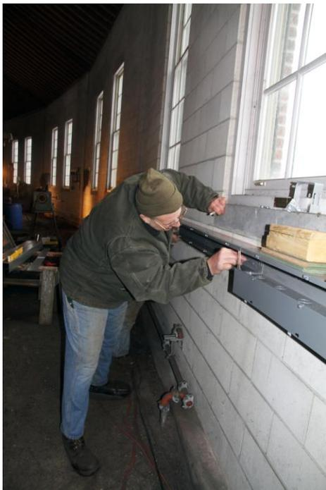
Steve Melady prepares to install a section of steel conduit for electrical system along back wall. (Robert A. LaMay Photo)
