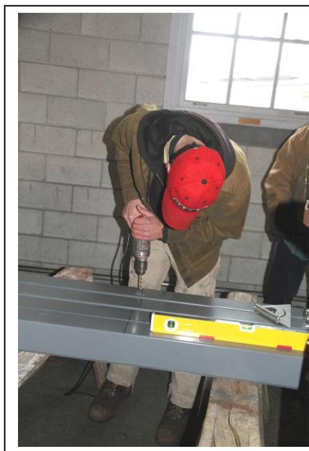
The photo at the bottom of the previous column shows Tom Schubert drilling holes in the steel conduit so it can be hung along the various walls. (Robert A. LaMay Photo)
