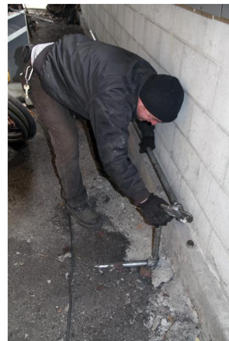
Shown here, Bill Voovart is installing piping for the compressed air system along the south wall in the roundhouse next to Pit number 1. (R. A. LaMay Photo)
