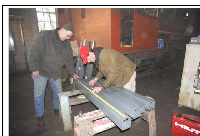
Steve Melady holds tape measure while Tom Schubert measures where to drill holes into the 4"x4" steel duct work which will hold the wiring for the new electrical system being installed in roundhouse. (Full story inside) (Robert A. LaMay Photo)
