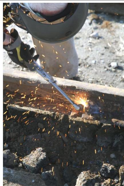
Shown here 'Torch' Hassett burns off the rusted and corroded nuts so the bolts can be safely removed. (Robert A. LaMay Photo)
