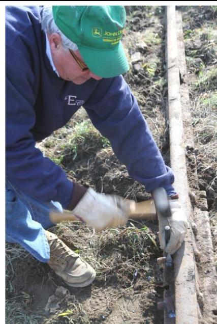
'Buster' Lund removes the pieces of burnt nuts so the bolts can be removed. (R. A. LaMay Photo)
