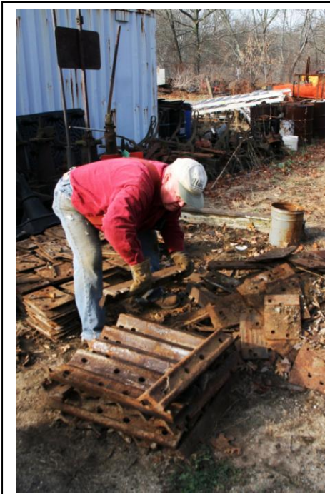
Adrian Atkins sorts joint bars and tie plates from the Mansfield Depot Rte 44 crossing job. (Robert A. LaMay Photo)
