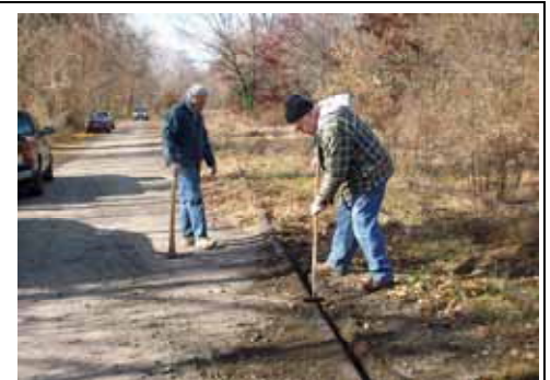
Cliff Lund (left) and Walt Dumas clear the flange-ways along museum driveway. (Jean Lambert Photo)
