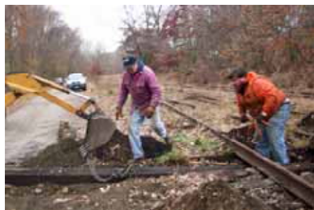
Rolf Johnson and Rich Cizik, Jr. help with the installation of a replacement tie. (Jean Lambert Photo)
