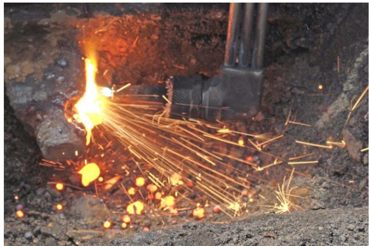
Close up of how to burn a rusted nut when removing old tie plates. (Robert A. LaMay Photo)
