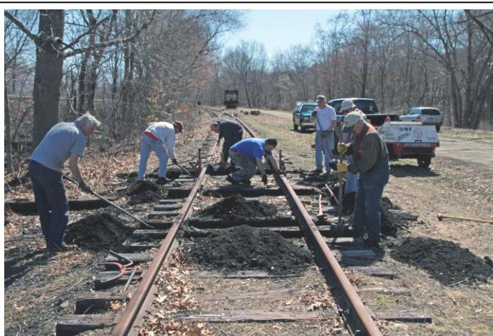
A large track crew works on the Air Line Route replacing numerous railroad ties. Keeping tracks safe for train rides is a necessity. It must be done prior to opening day. (LaMay Photo)
