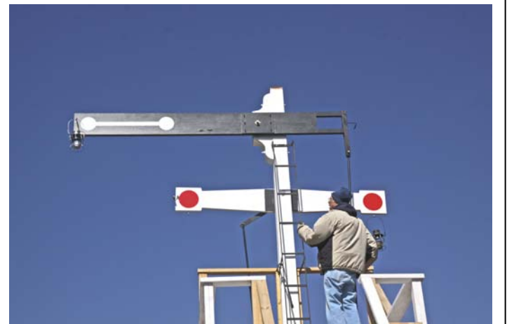
Dick Arnold checks clearances with lanterns on the Gallows Signal's moveable arms. (Robert A. LaMay Photo)
