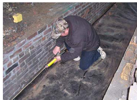
Bill Voorvaart completes the sealing process of the liner in Pit number 2. (Adrian Atkins Photo)
