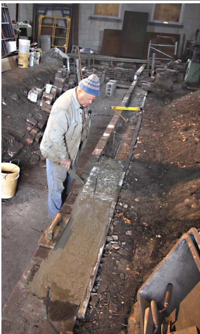
Adrian Atkins works in smoothing the new concrete being poured during the rebuilding and reconstruction of Pit no. 2. (Robert A. LaMay Photo)
