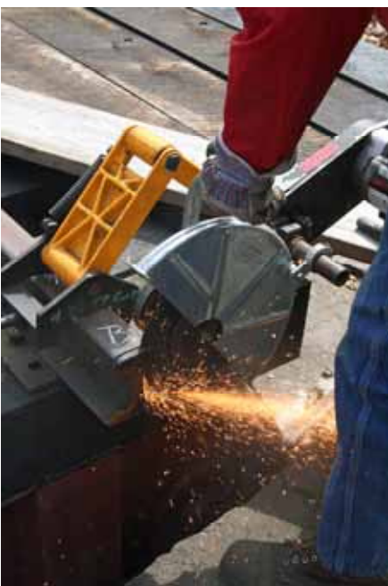
The sparks fly as our rail saw cuts through a piece of rail on turntable bridge. (Robert A. LaMay Photo)
