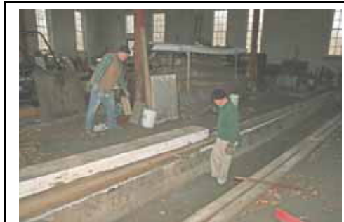
Walt Dumas and Duke York get ready to move timbers into position in Pit No. 4. (Robert A. LaMay Photo)
