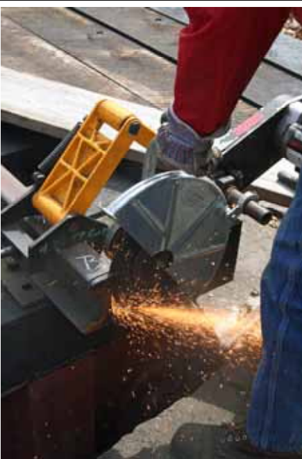
The sparks fly as our rail saw cuts through a piece of rail on turntable bridge. (Robert A. LaMay Photo)
