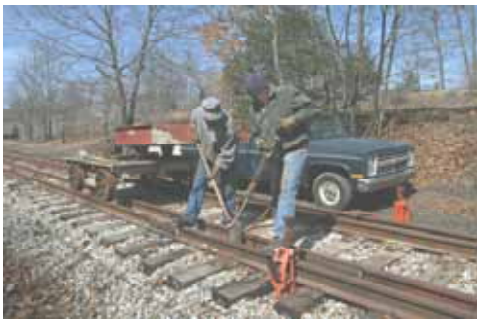
Mark Granville spreads ballast as Art Hall, Jr. tamps around one of the museum's switches. (Robert A. LaMay Photo)
