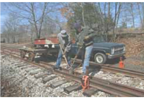
Mark Granville spreads ballast as Art Hall, Jr. tamps around one of the museum's switches. (Robert A. LaMay Photo)
